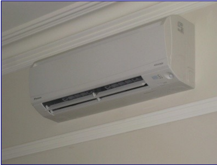
Figure A4.9: Reverse-cycle air conditioner
