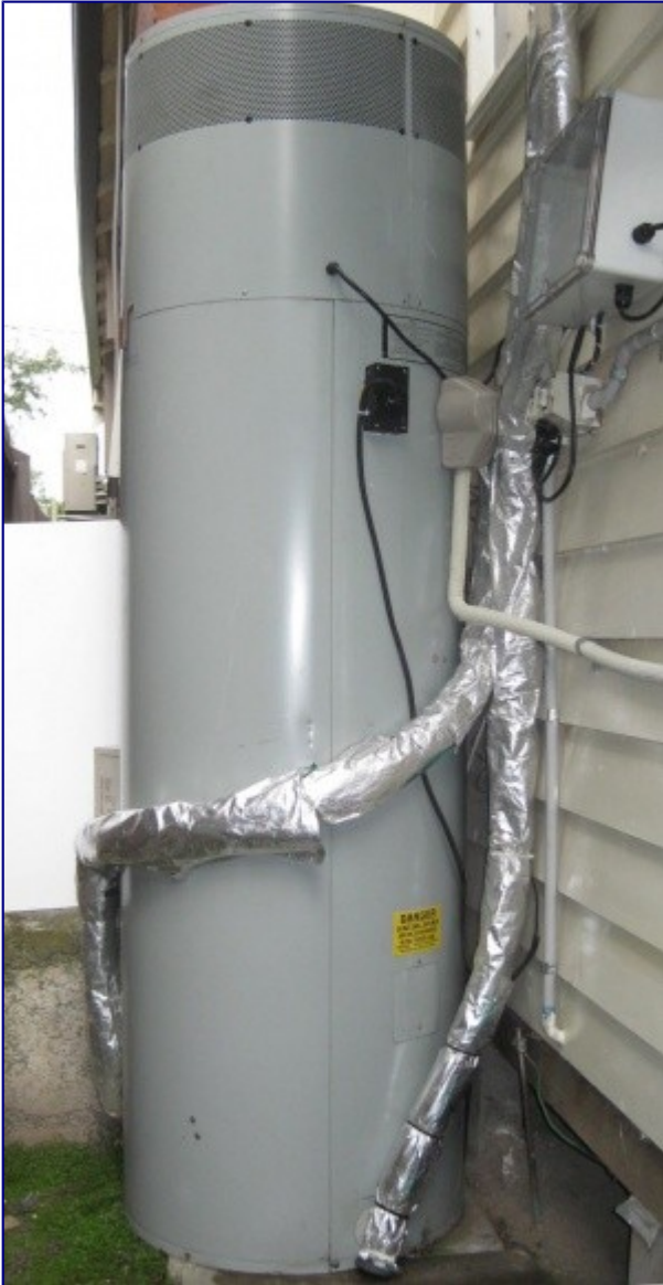
Figure A4.6: Heat pump hot water unit
